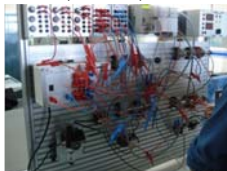
电气(PLC)回路搭接
